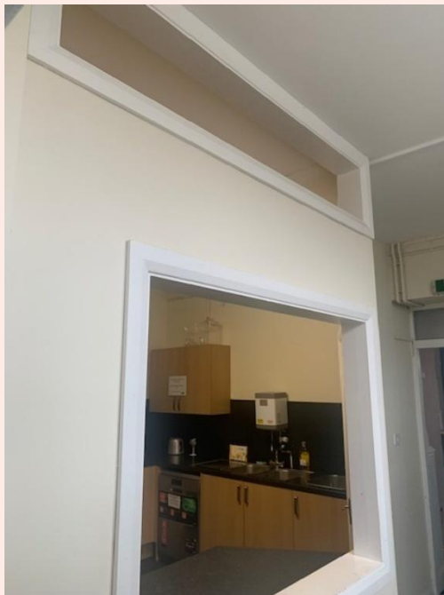
Showing open hatchway and top of wall vision panels
