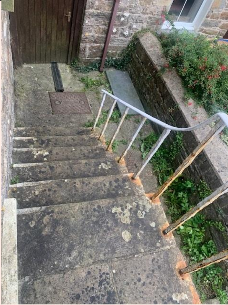
Rear final exit route
