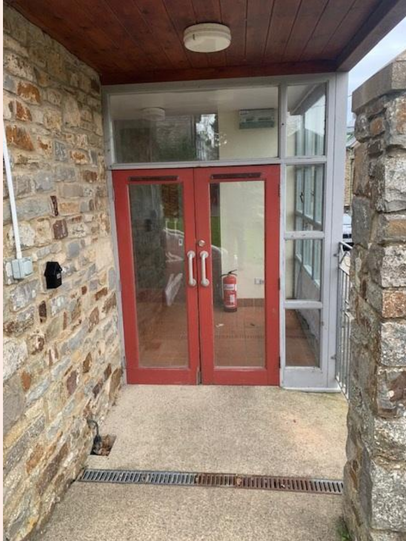
Main entrance and hallway
