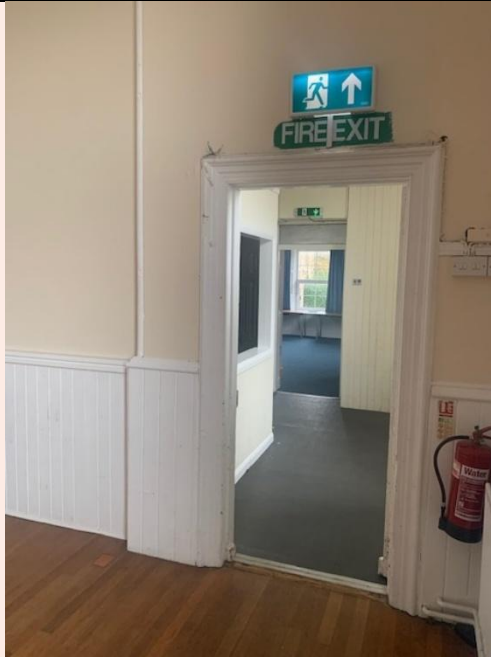
Doorway from main hall into kitchen and meeting room
