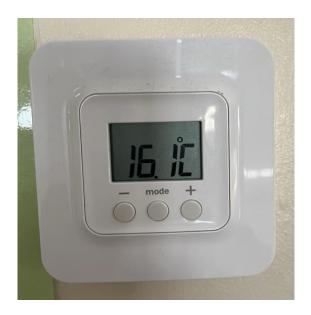
ONLY USE THE MIDDLE BUTTON. To switch on press middle button until "ON" is displayed on top left of screen:
